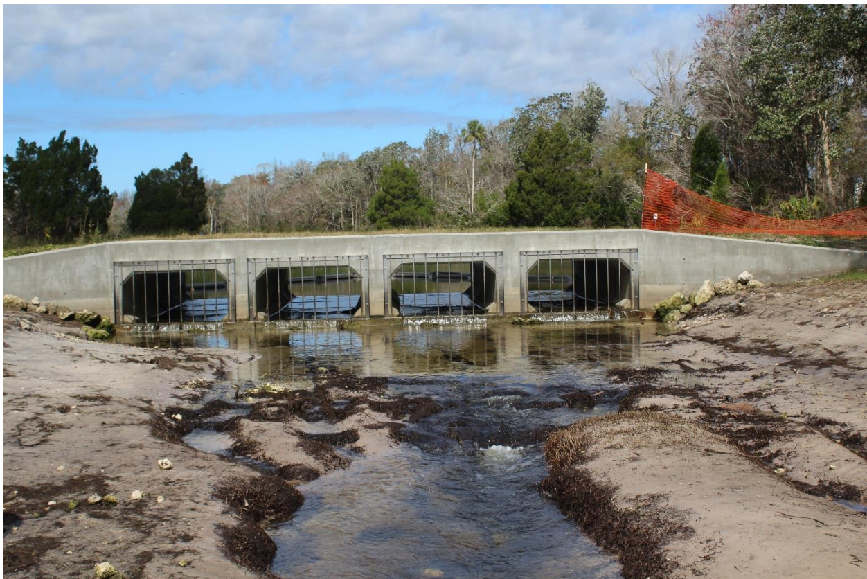
Photo of manatee exclusion grates on box culverts at Crystal River National Wildlife Refuge.
