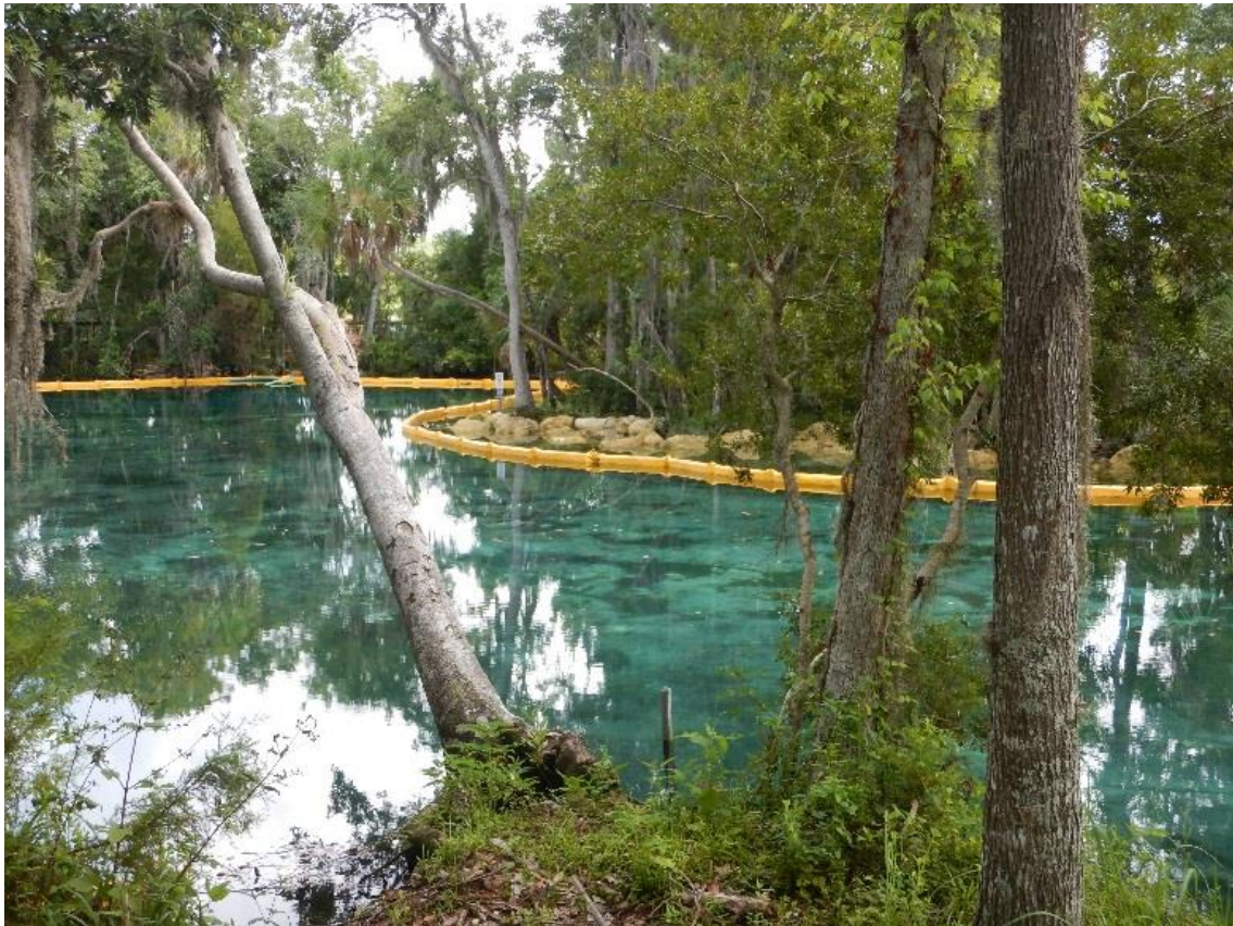
Photo of Three Sister's Springs shoreline stabilization project. (Citrus County).
