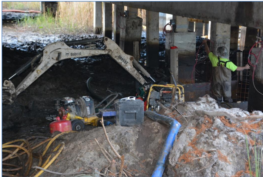
Work under I-95 at Little Cedar Creek Bridge
