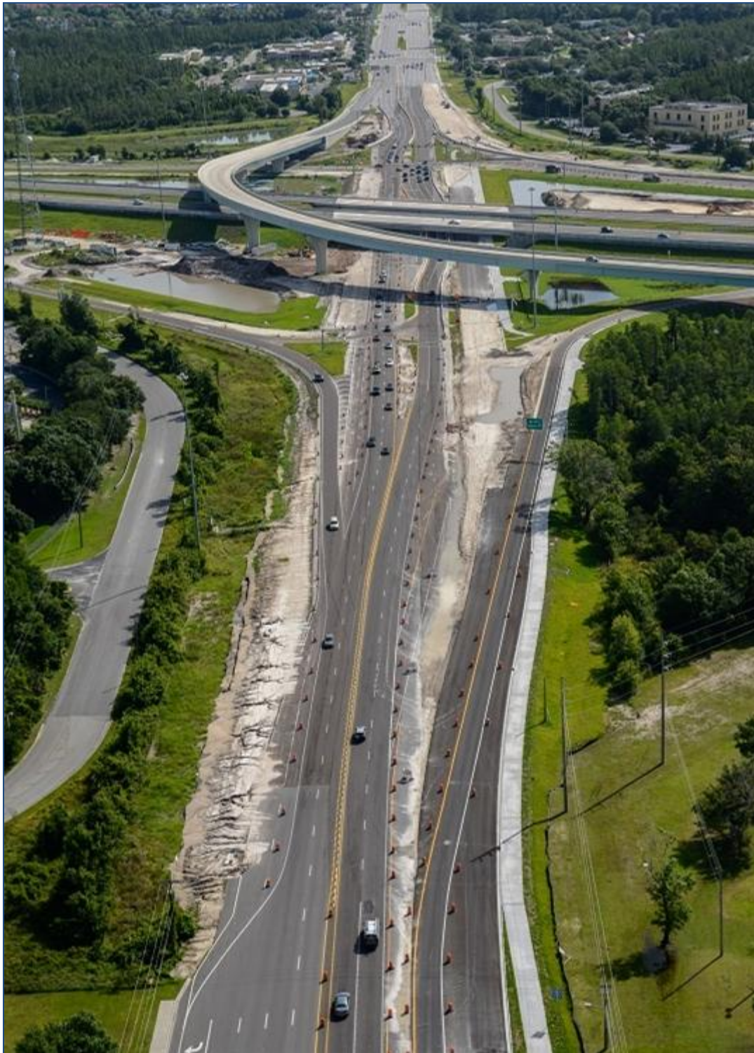
Widening Bruce B. Downs Blvd at I-75 Interchange
