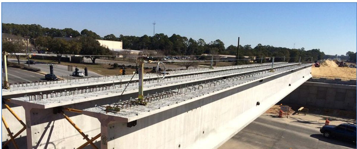
Beams set on US 98 and Cody Avenue- Okaloosa County
