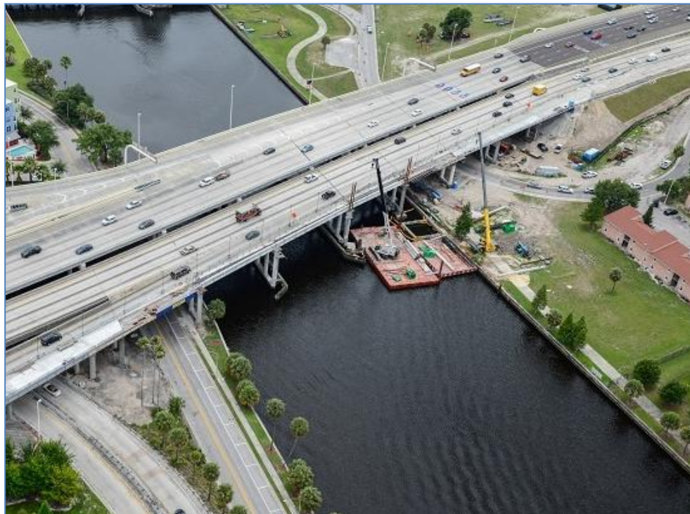
Bridge widening downtown Tampa
