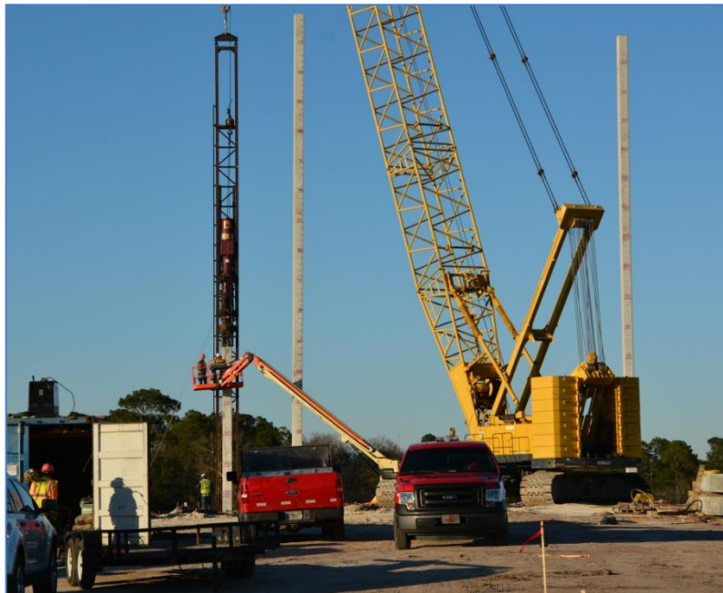
Pile driving I-10 and Hammond
