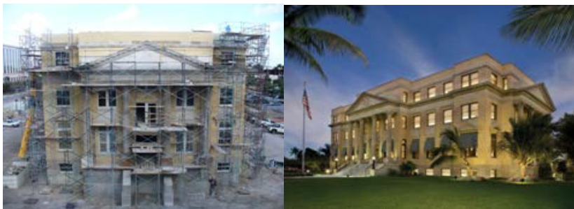
Figure 3 - Historic 1912 Palm Beach County Courthouse Restoration Before and After
