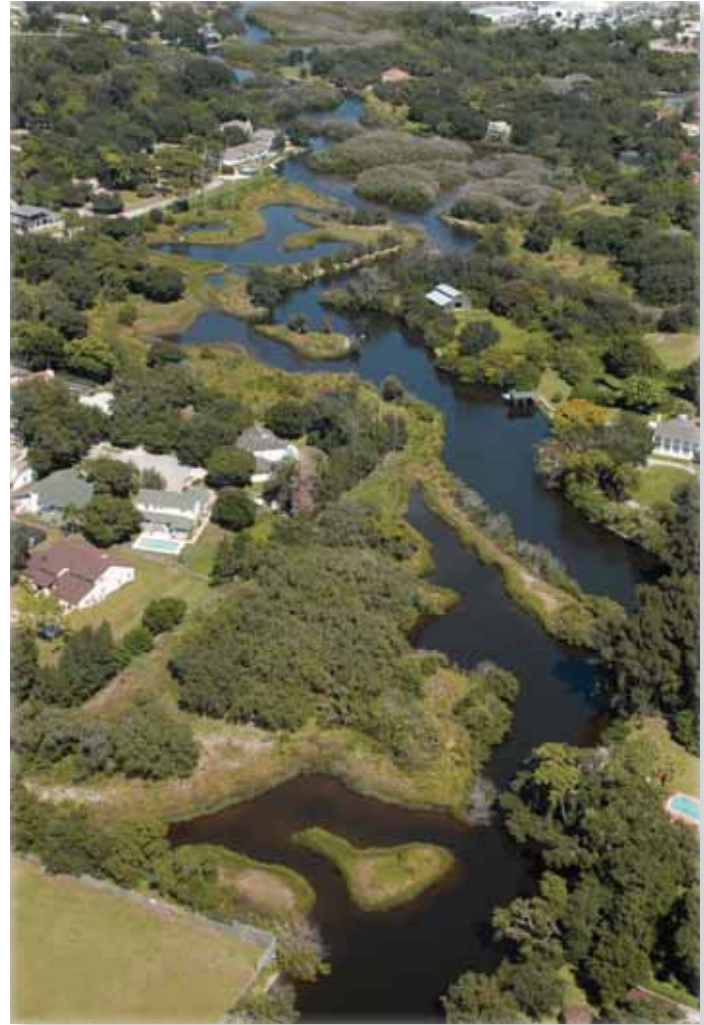
Lancaster Tract Restoration Project created several new wetland areas and also formed a freshwater pond to collect and treat stormwater entering the site. Lancaster Tract now provides improved water quality entering Tampa Bay.
