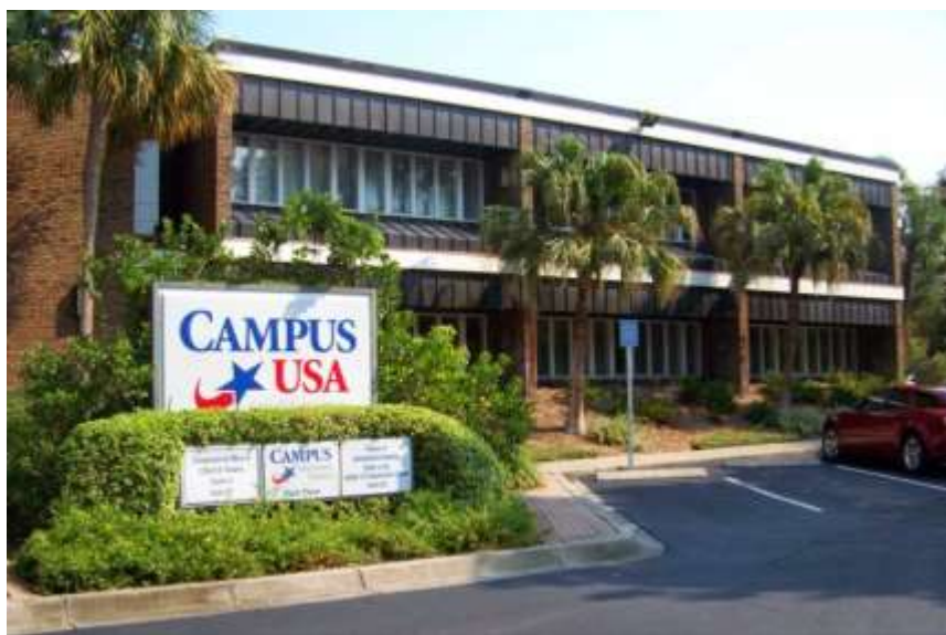
Gainesville District Office on West 34 th Street
