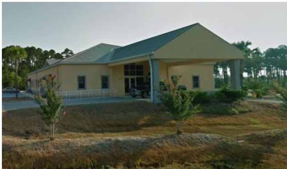
Panama City District Office on State Street and 23 rd Circle
