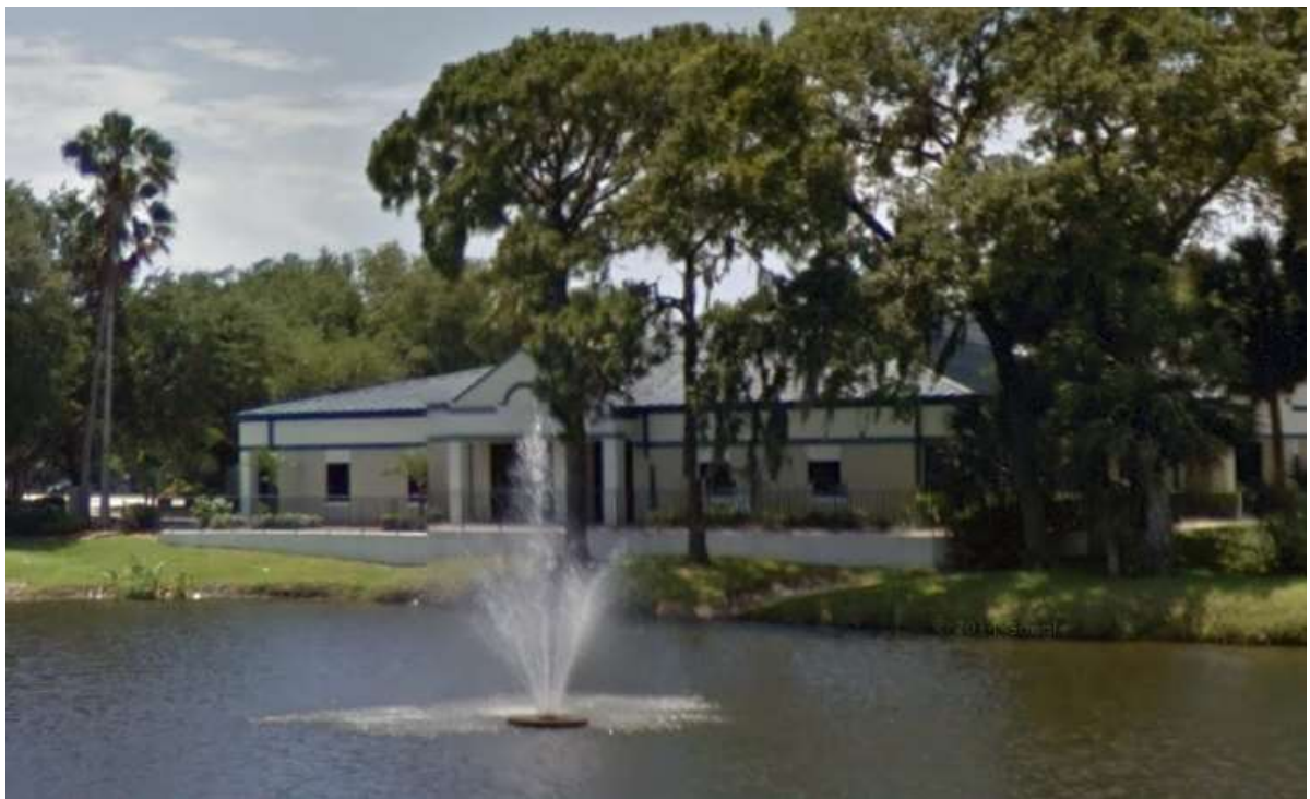
Sarasota District Office on Parkland Drive
