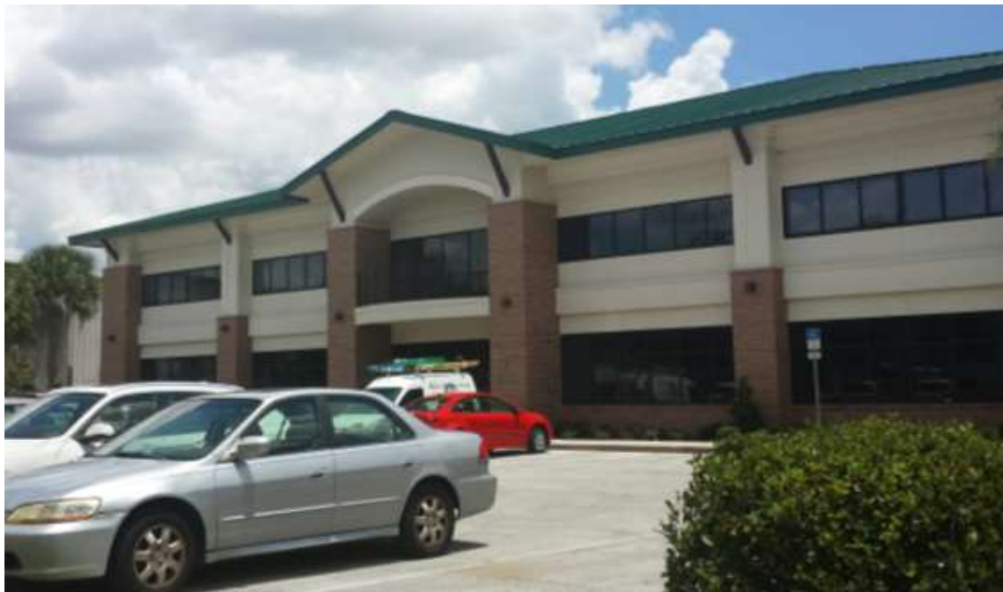
The new Lakeland District Office. A welcome change for central Florida.
