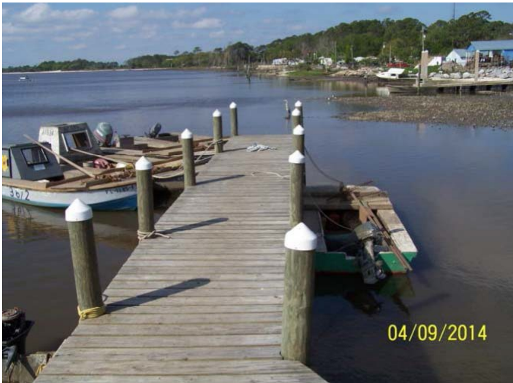
The end of the existing dock showing the oyster boats tied up. The tall concrete pilings in the right background are at the county boat ramp.
