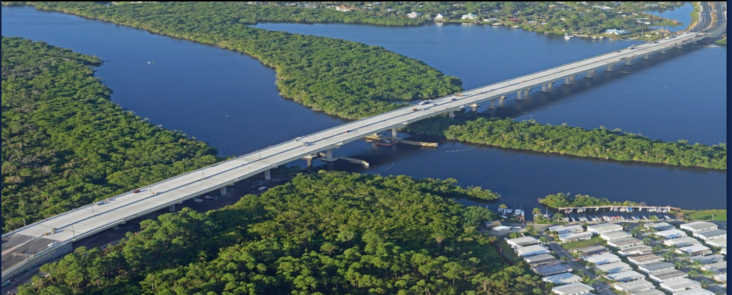
Veterans Memorial Bridge - Photo courtesy of www.seefloridago.com
