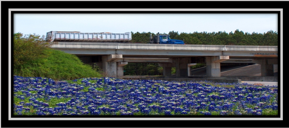
District 2 - Photo courtesy of www.seefloridago.com
