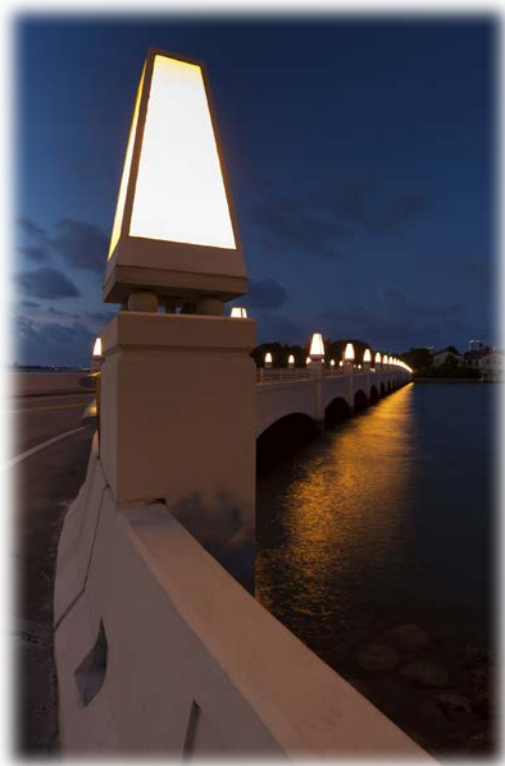
Star Island Bridge connects to a man-made island in Biscayne Bay, Florida.
