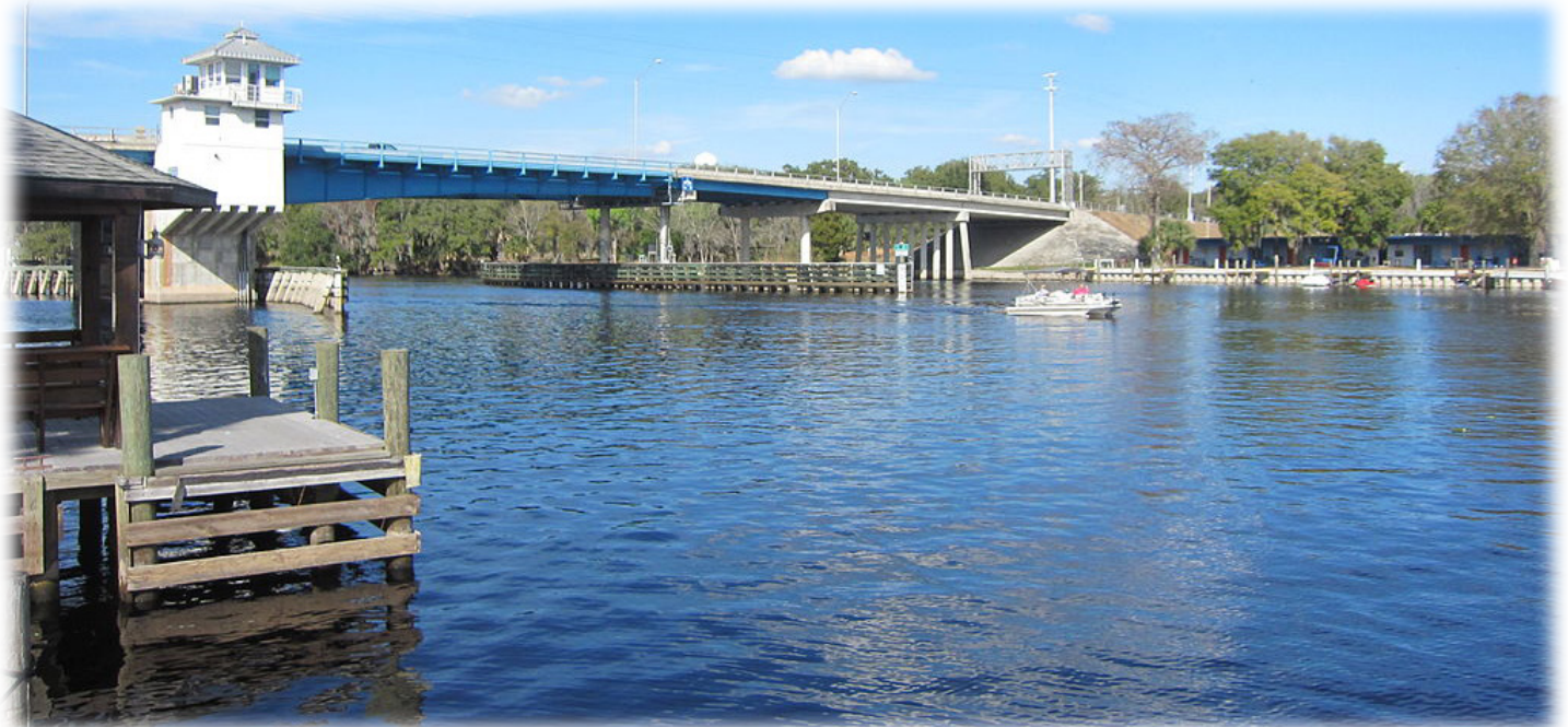
Astor Bridge is a single-leaf bascule bridge located in Astor, Florida that carries State Road 40 over the St. Johns River
