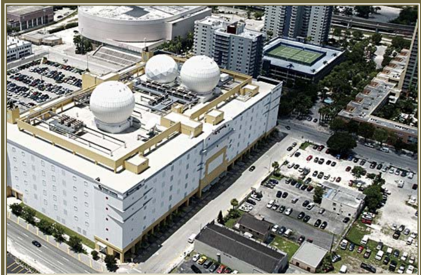
Network Access Point of the Americas in Miami - Terremark Building. Alternative site for IT Infrastructure Systems.
