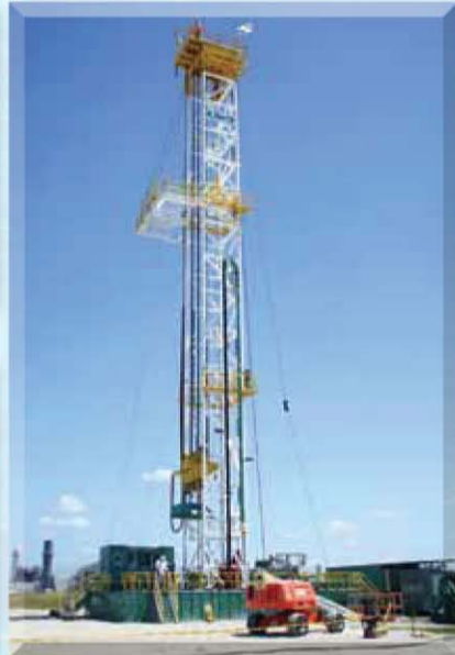
TECO Drill Site
