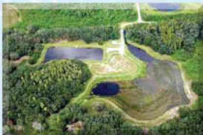
Eastshore Commerce Park Stormwater Hillsborough Co.
