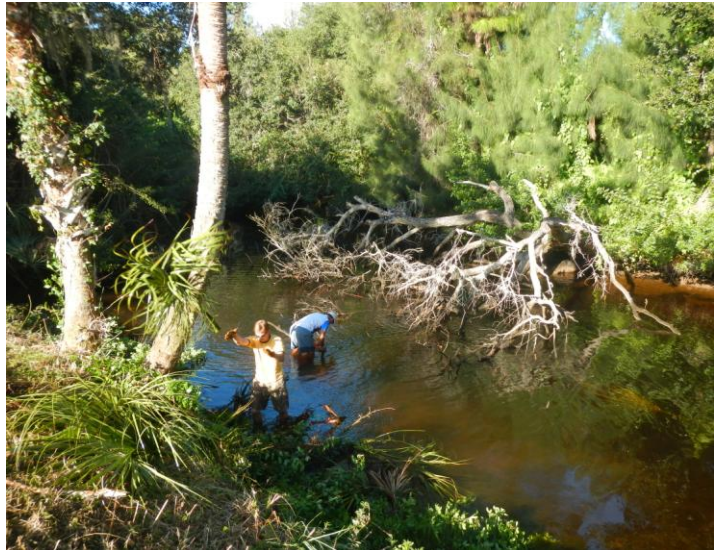
Debris removal in Salt Creek to improve manatee access.
