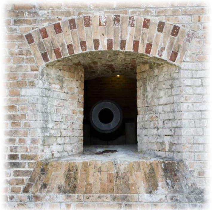
U.S. Civil War cannon embrasure at Fort Pickens, Gulf Islands National Seashore.
