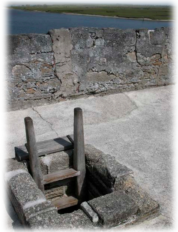
Fort Matanzas roof hatch to fort rooftop in St. Augustine, Florida.
