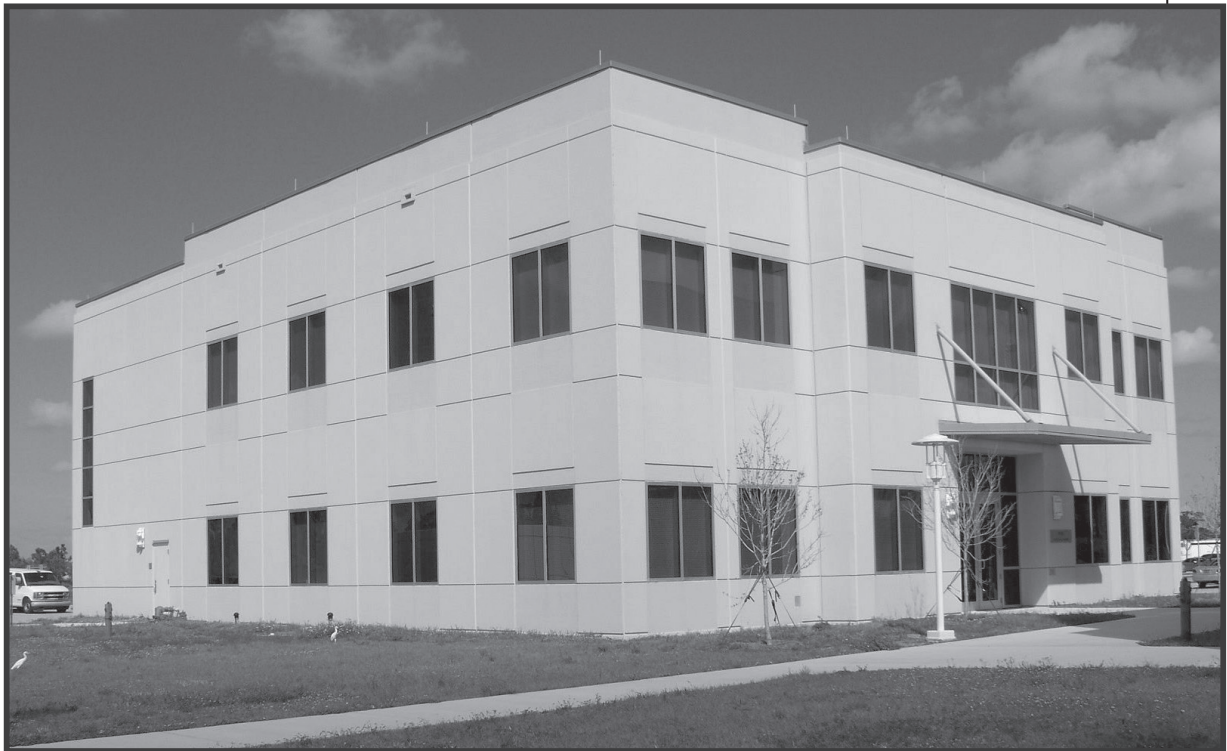
Department of Highway Safety and Motor Vehicles - Florida Highway Patrol Office Building - Palm Beach County
