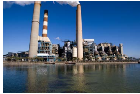
TECO Big Bend Power Station
