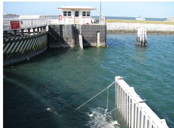
Repairs to Canaveral Locks
