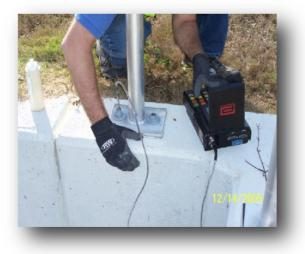
Nondestructive ultrasonic testing was used to verify whether the anchor bolts installed by Almar met department design specifications
