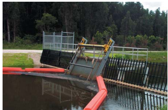
Water-control structure, Miami-Dade County.
