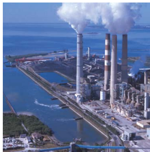
TECO's Big Bend power plant and discharge canal, located in Apollo Beach.
