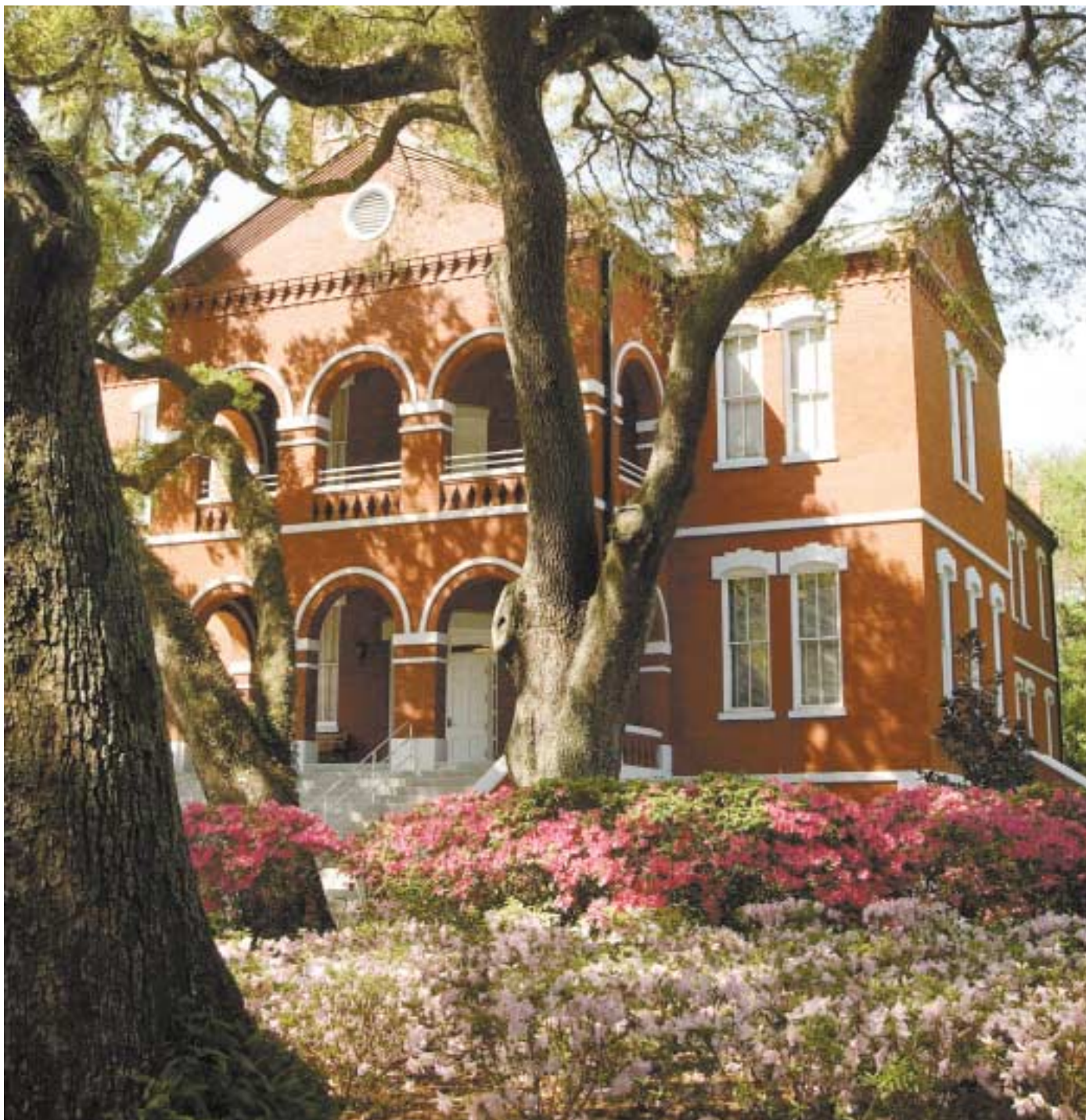
Almost 800 local governments in Florida benefit from the SBA's experience in managing and investing surplus funds on their behalf. (above: Osceola County courthouse, the oldest courthouse in continuous use in Florida)
