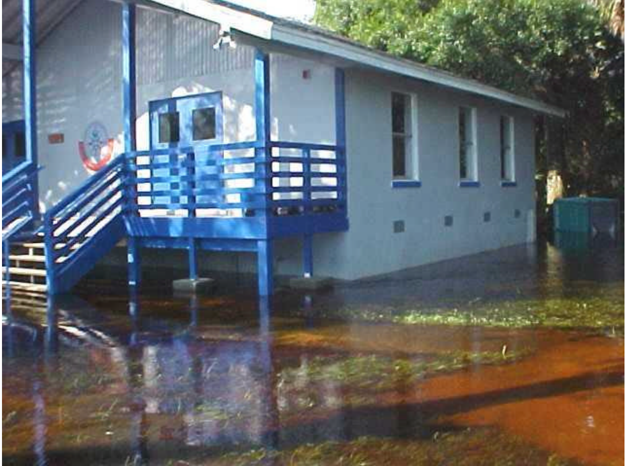
Heavy rains caused flooding at State-owned Myakka Park in Central Florida
