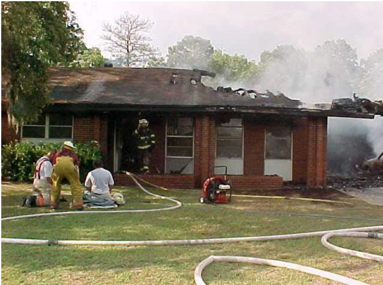
State owned residence severely damaged by fire in Sumter County
