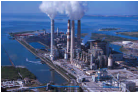
Tampa Electric Company's Big Bend power plant
