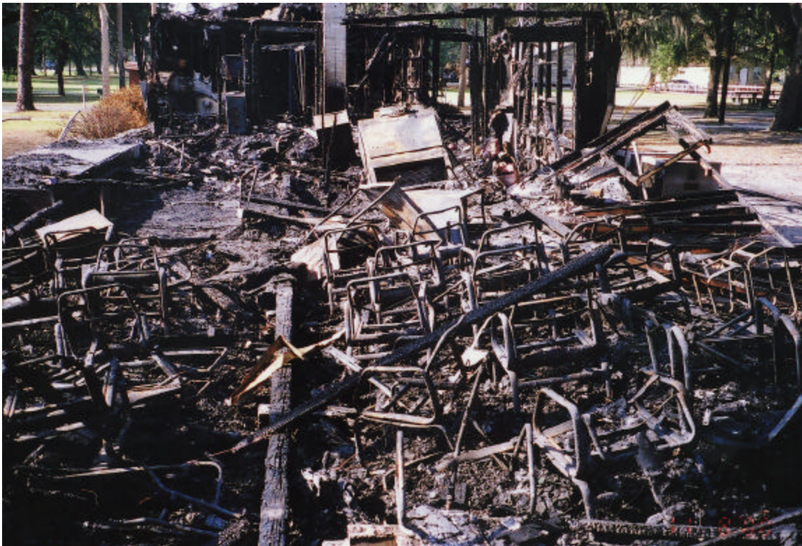
Fire destroys State owned building and contents in Desoto County
