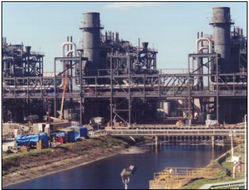
Fort Myers Power Plant - The plant was recently re-powered extending its life at least 30 years. A manatee protection plan assured that manatees were not harmed during the transition.
