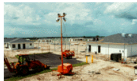
Wilderness Camp under construction.
