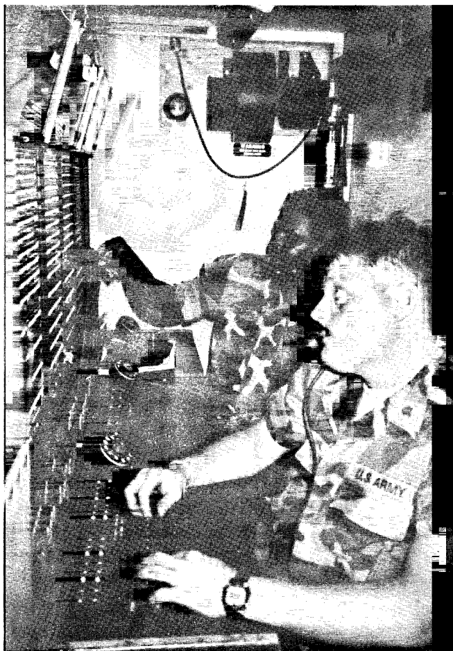
Troops from 653rd Signal Company operate switchboard
