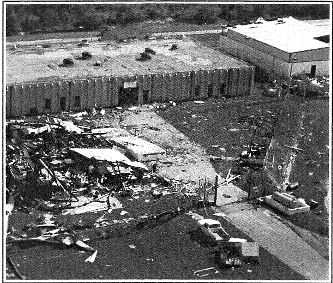
Hurricane Andrew damaged or destroyed most of Dade C.I. and Dade Work Camp. The Office of Operations was instrumental in evacuating these facilities and coordinating the transfer of inmates to nearby prisons.
