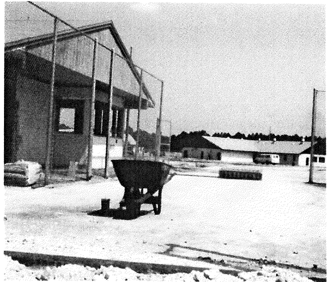
Construction at Gainesville Drug Treatment Center.
