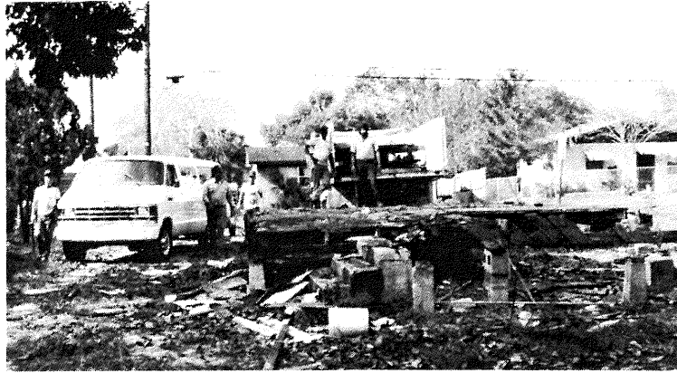
Inmate Work Squad demolishes a "crack house" in Tarpon Springs.
