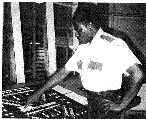
Correctional Officer works the central panel to lock-down individual cells during "count."
