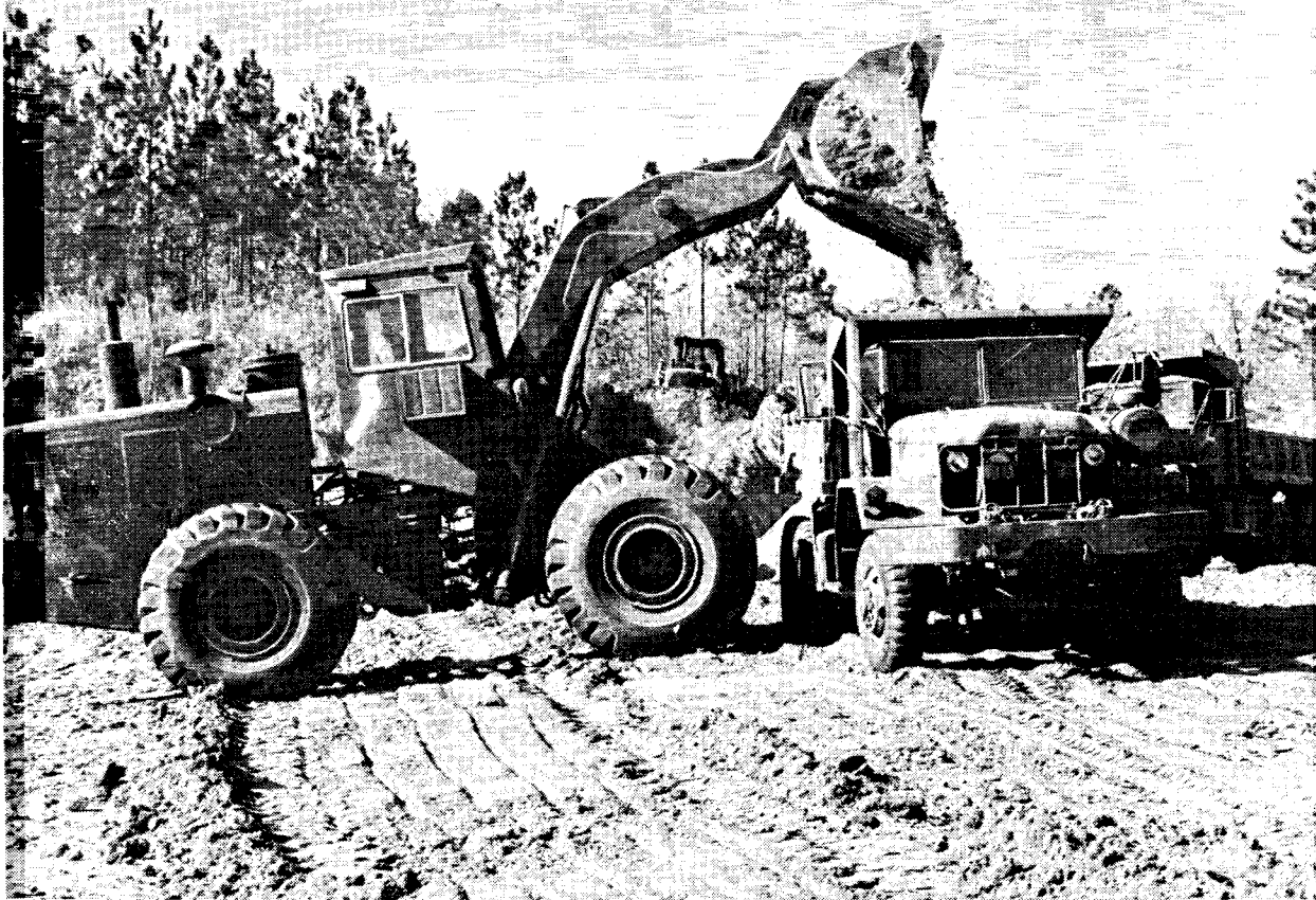
Engineers perform construction at Camp Blanding
