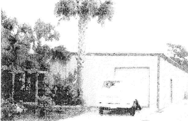
Warehouse expansion of PRIDE's printing plant at Zephyrhills C.I.
