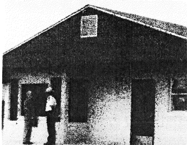
The control room of Hendry C.I.'s "Farm Camp."
