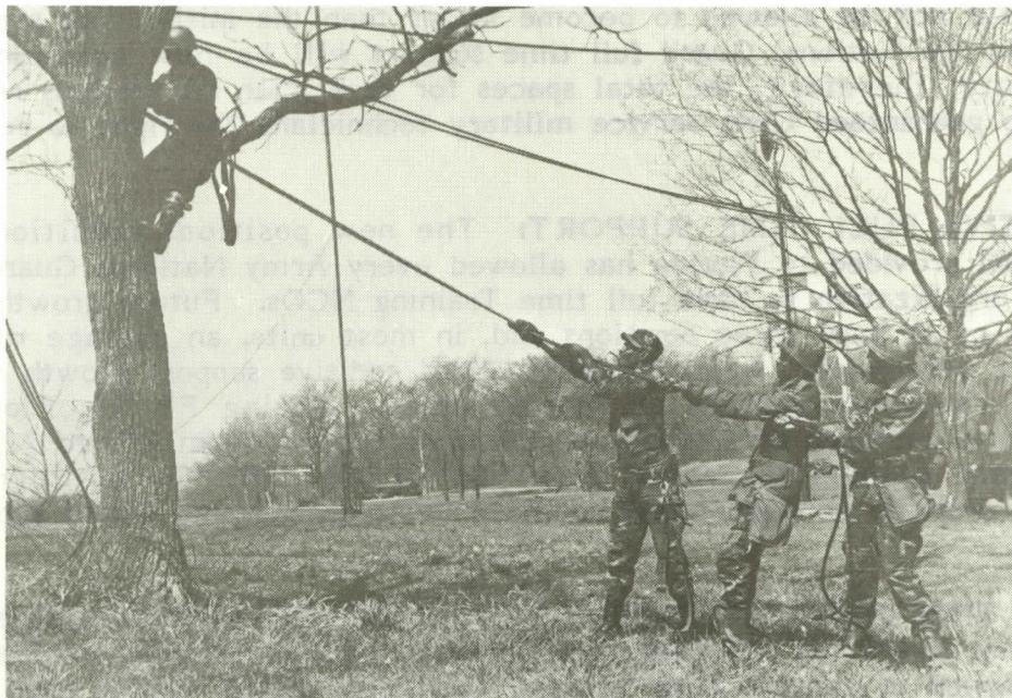
Soldiers of the 146th Signal Battalion pull wire "overhead"
