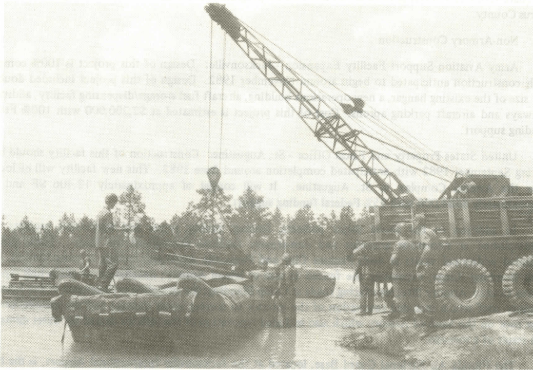
Engineer Unit trains with bridging equipment at Camp Blanding, Florida
