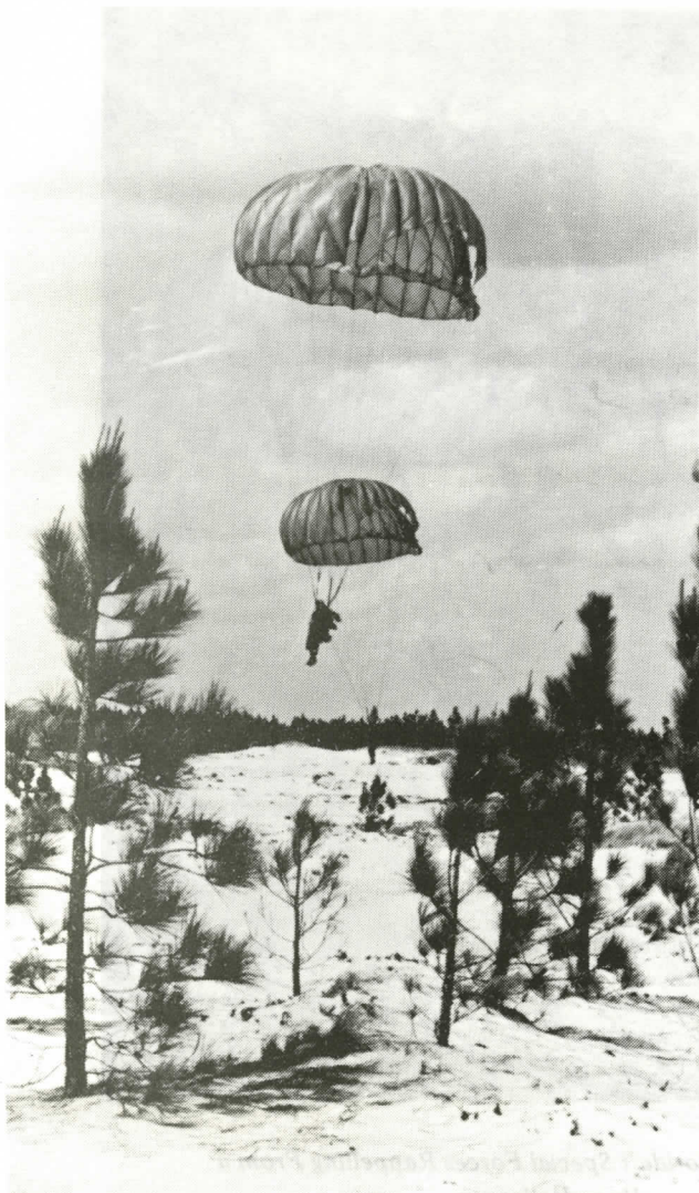
One of the Two Approved Drop Zones in Operation at Camp Blanding.
